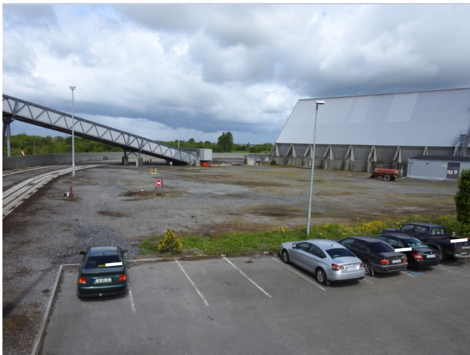
Figure 4-8: Ground view of Biomass Storage Slab A
